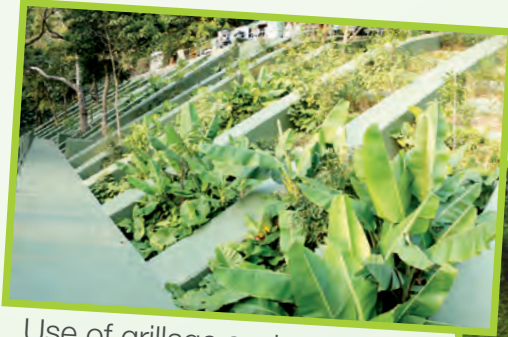
Use of grillage system to retain existing vegetation
