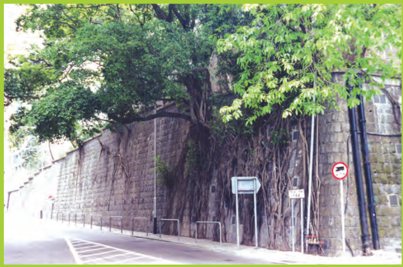
Existing wall trees are retained after upgrading works using soil nails
