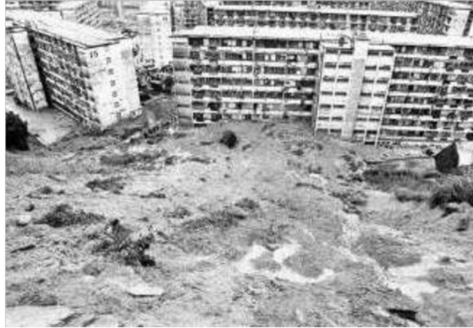
Figure 3: Sau Mau Ping Landslide in 1976 (resulting in 18 fatalities)
