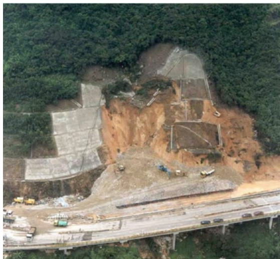
Figure 6: Ching Cheung Road Landslide in 1997 (~5,000m 3 )
