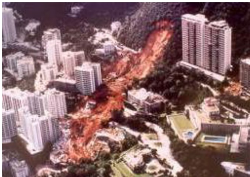
Figure 2: Po Shan Landslide in 1972 (resulting in 67 fatalities)
