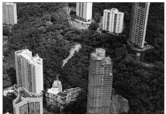
Fig. 2. A relatively modest 50 m 3 landslide in 1998 had resulted in damage to property
