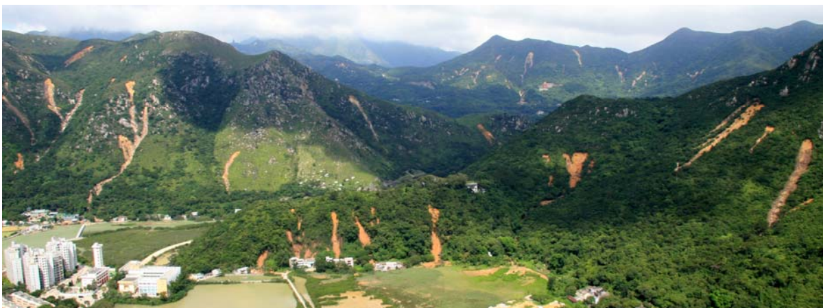
Fig. 19. Example of landslide clusters in West Lantau from the June 2008 rainstorm
