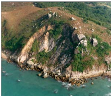
Fig. 6a. Large coastal landslide on Lamma Island
