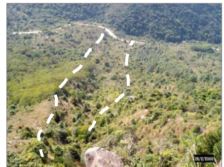
Fig. 6c. Large relict landslide above Tung Chung Road, Lantau Island
