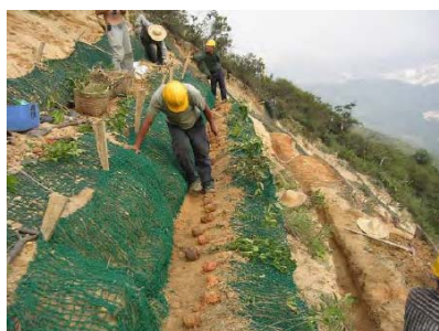
(b) Laying out rooted plants for hedgelay installation
