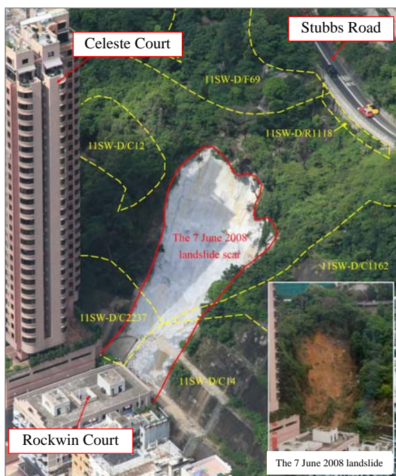
Fig. 27. Examples of failures within hillside pockets
