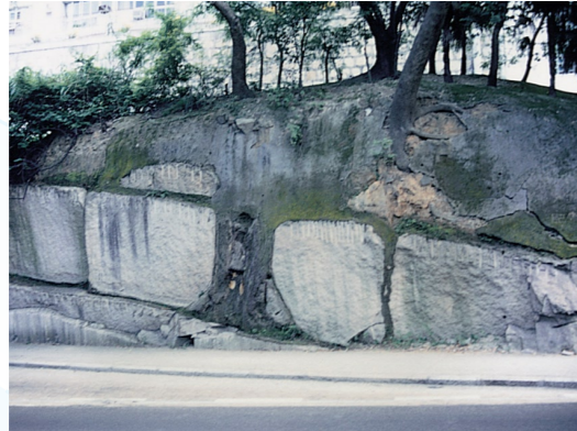
圖1. 花崗岩中的垂直節理受風化而變寬。 Figure 1. Vertical joints in granite widened by weathering.
