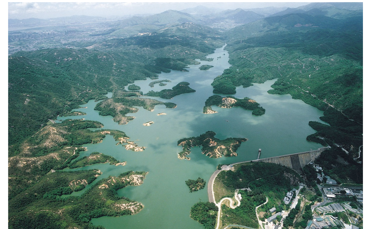
圖2. 沿大欖斷層侵蝕而成的筆直河谷。 Figure 2. Linear valley eroded along the Tai Lam Fault.
