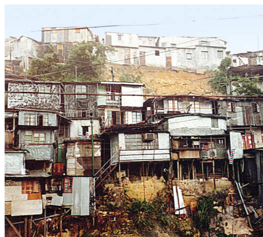
圖27. 用一般工程方法不能有效處理寮屋斜坡問題。 Figure 27. Engineering works approach is normally not an effective way to deal with slopes with squatters.
