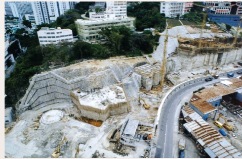
圖4. 建造樓宇時要切割大量山坡。 Figure 4. Building platforms are formed by cutting into the hillside.
